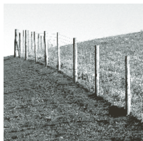
Example of pig netting fencing.
