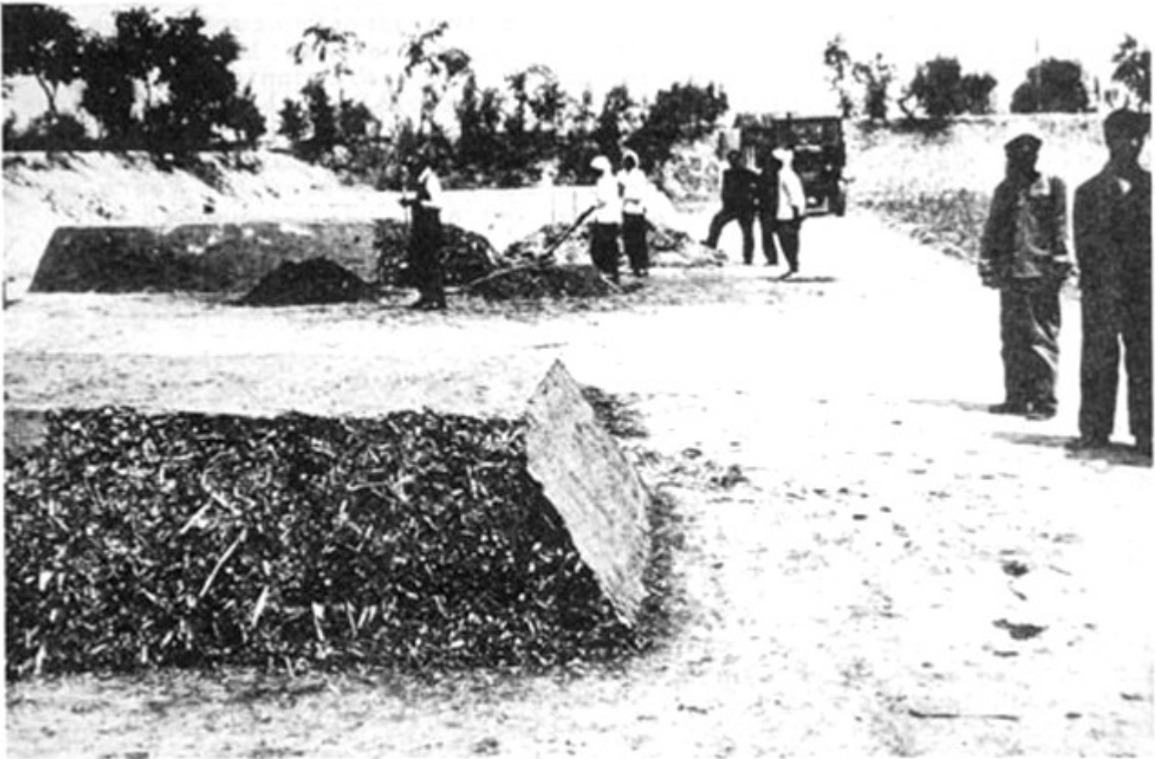
Plate 17 Chinese high temperature heap, mud covering in place on sloping sides; this holds in the heat and odours and prevents fly breeding Source: FAO (1978c)
