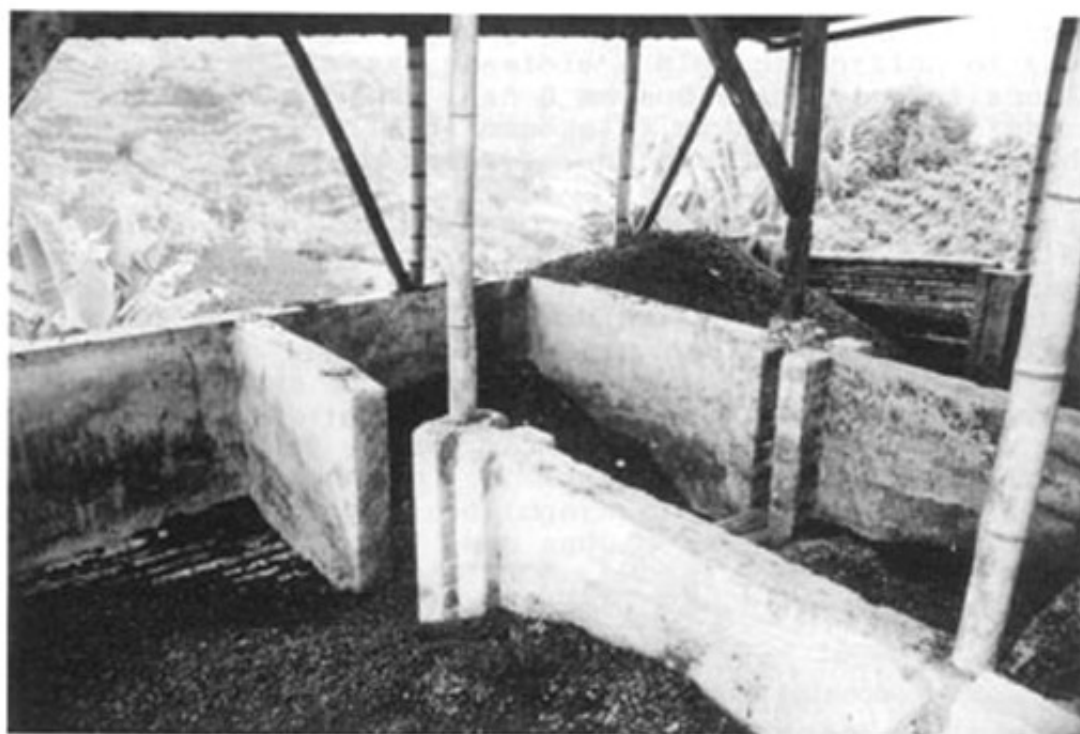
Plate 18 Compost pit on coffee estate with side walls, overhead cover and perforated floor for aeration Source: FAO filmstrip Uses of Coffee Pulp
