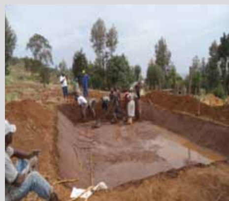
Mud is spread (left), a thin mud paste is smeared and water added to avoid cracking (right).
