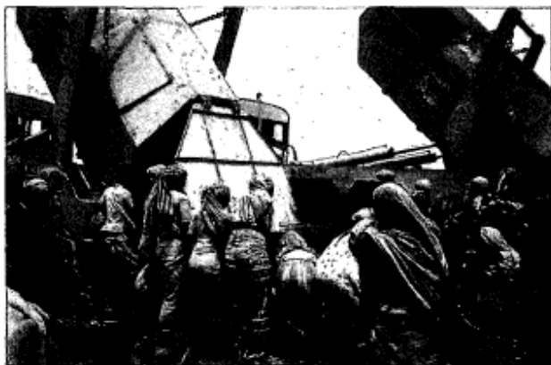
Photo: WASTE Consultants, 1991
