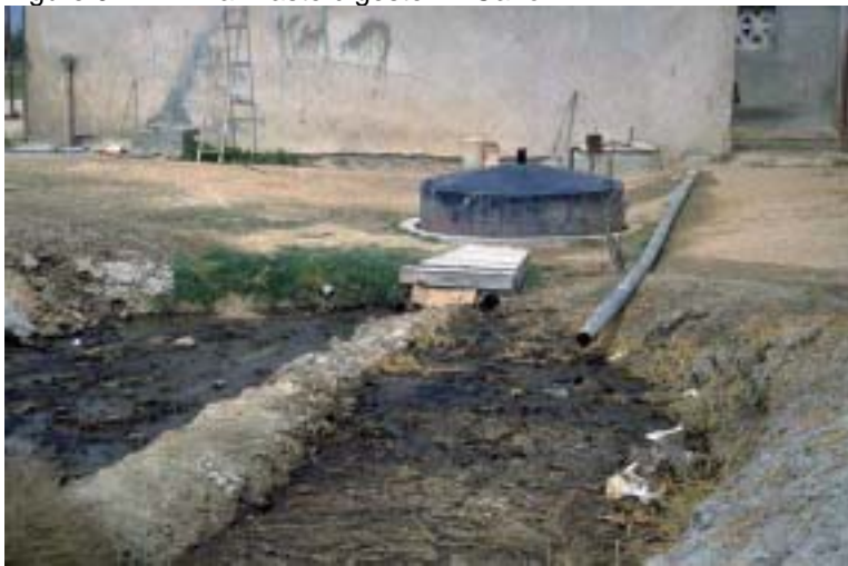
Photo: WASTE Consultants, 1993.
